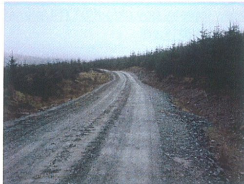
6. Looking North back along C262
